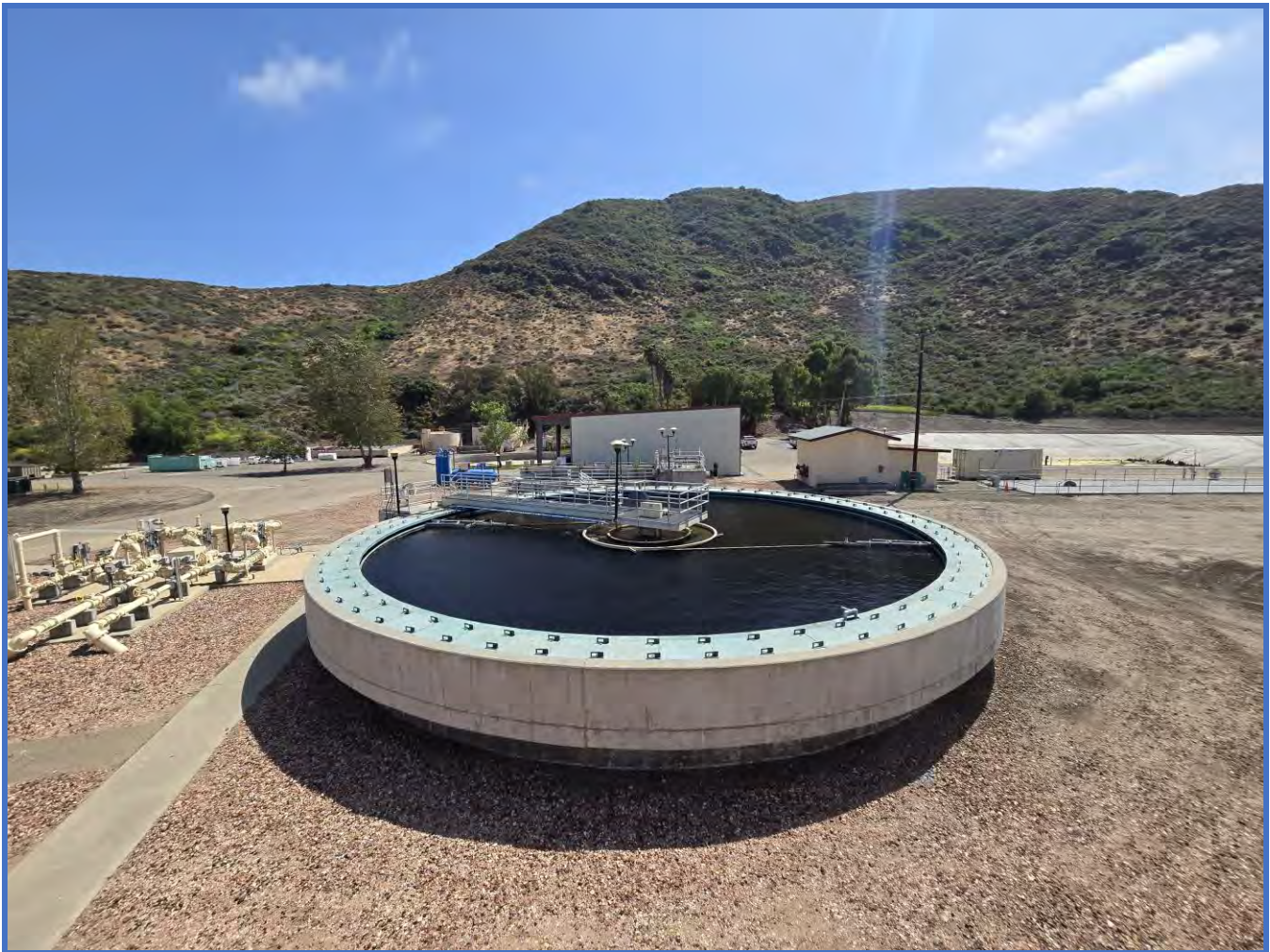
Camrosa Wastewater Reclamation Facility Clarifier
