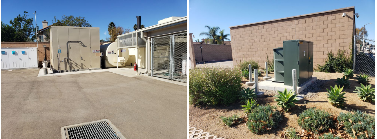
Figure 3 – Existing Lynwood Well Site at Woodcreek Park
